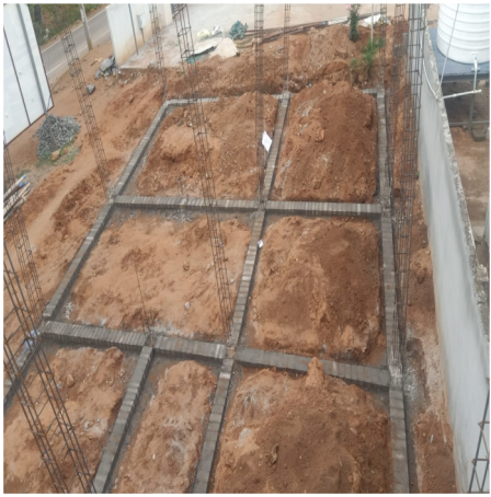
Basement Belt Laying
