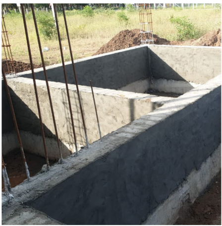
Basement Inner Plastering
