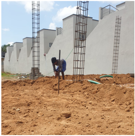
Belt Beam Concrete
