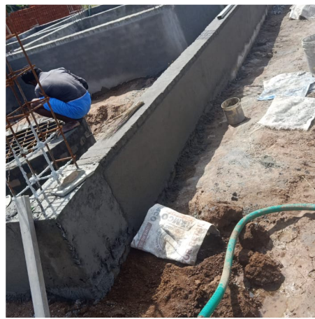
Basement Outer Plastering
